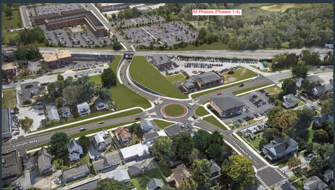
Source: City of Valparaiso Campbell Street – Lincolnway to Brown Street Construction Project
