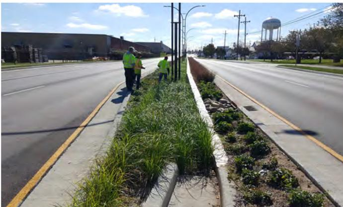
These images to the left portray the center median rain gardens. Features such as rip-rap at the location where water enters (image above) will help to collect any garbage and sediments to help reduce maintenance and increase plant survivability. A 12-18" maintenance zone of gravel could also be added around the perimeter to allow workers a safe area to stand out of the roadway while performing maintenance.
