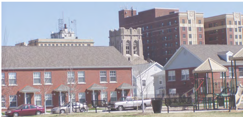
Horace Mann Hope VI residential project in downtown Gary. Photo courtesy of the city of Gary.
