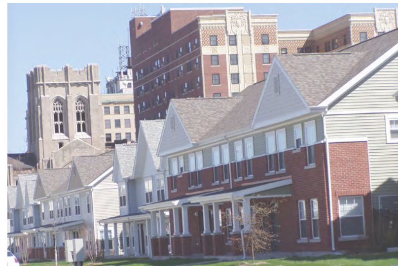
Horace Mann Hope VI Residential Project in downtown Gary. Photo courtesy of the city of Gary.
