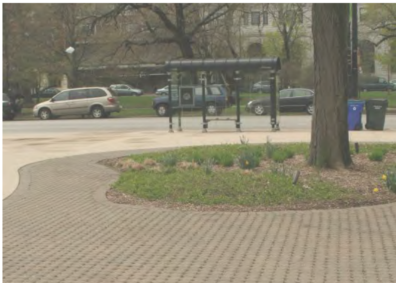
Permeable pavers in Chicago's Lincoln Park. Photo by Kathryn via Flickr.
