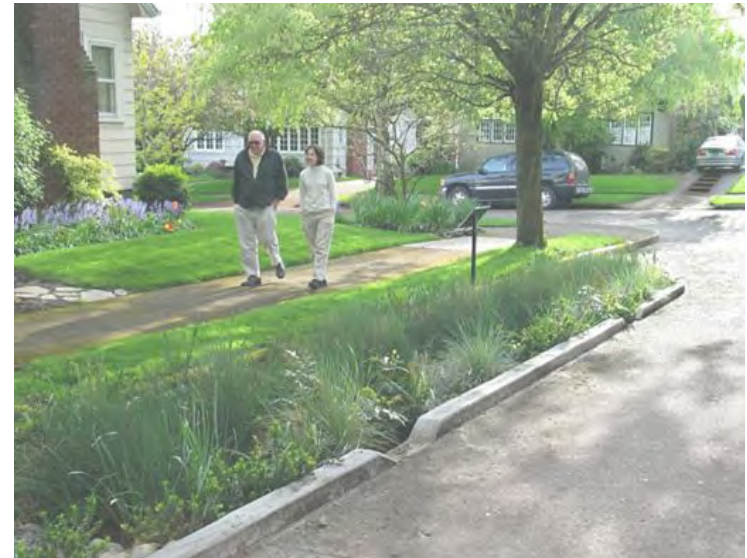
Curb cuts let stormwater into a roadside infiltration basin on a residential street. Photo from web.
