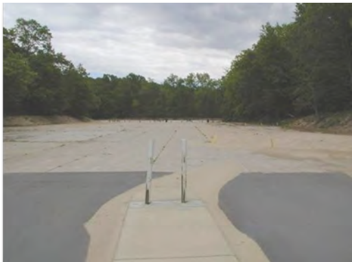
Dunes Creek before daylighting.
