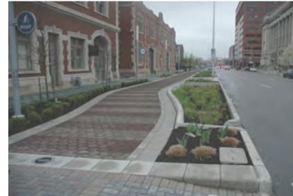
Constructed bioswale adjacent to urban street
