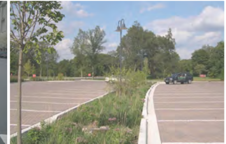
Constructed bioswale in parking lot
