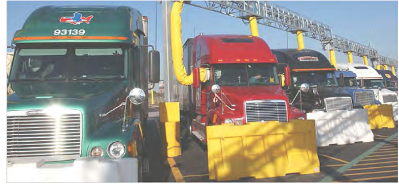
Tractor trailers plugged in at EPS in San Francisco. Photo from nytimes.com.
