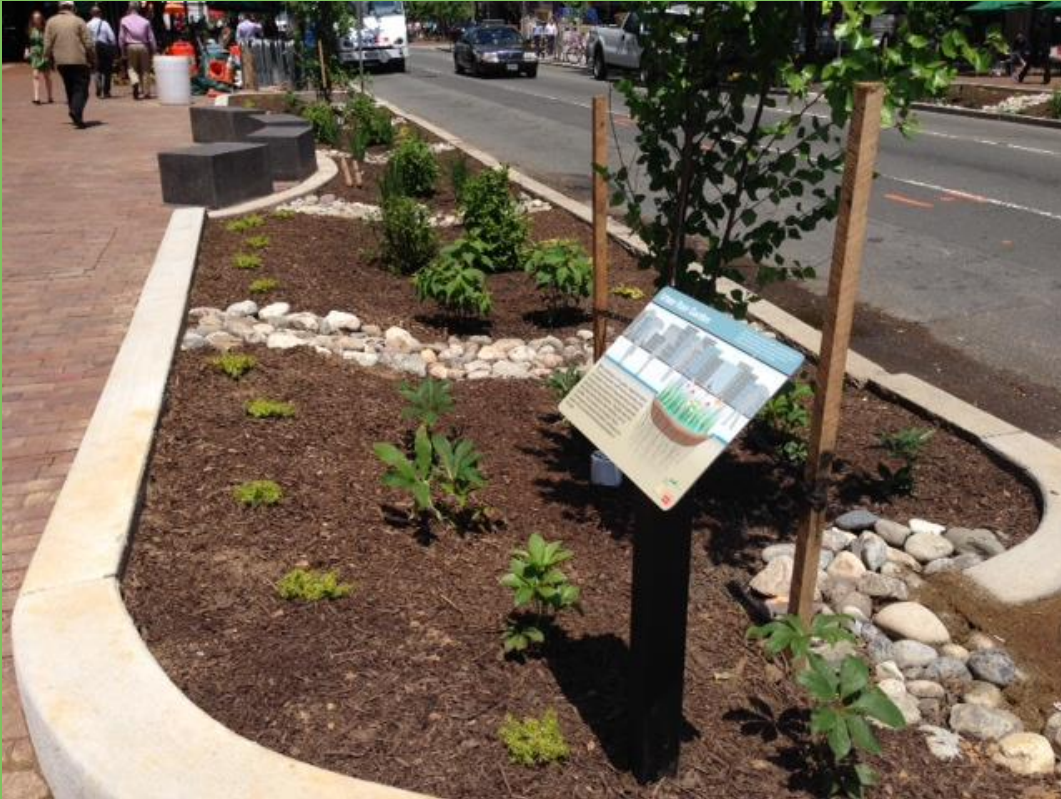
Rain garden infrastructure
