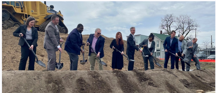
The RDA joined with local, state and federal officials in March 2024 to break ground for the new parking garage and station at 11th Street in Michigan City.
