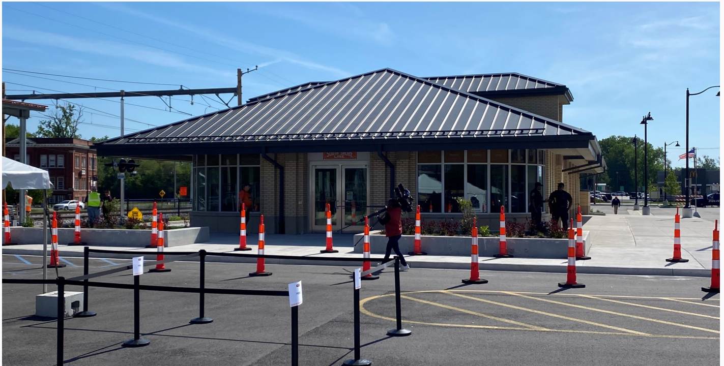
The new South Shore station in Miller. Featuring indoor seating, restrooms and space for retail, the station is a significant upgrade over the previous station. The project also included an upgraded and expanded parking lot.
