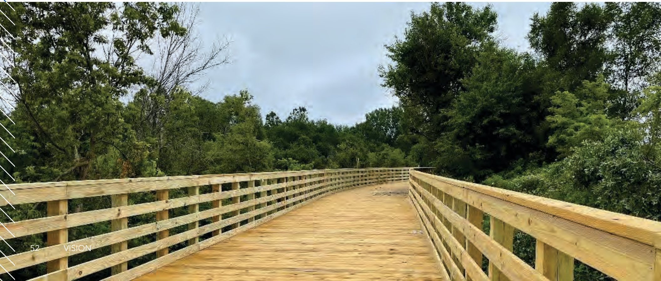
School Trail Bridge over Potato Creek
