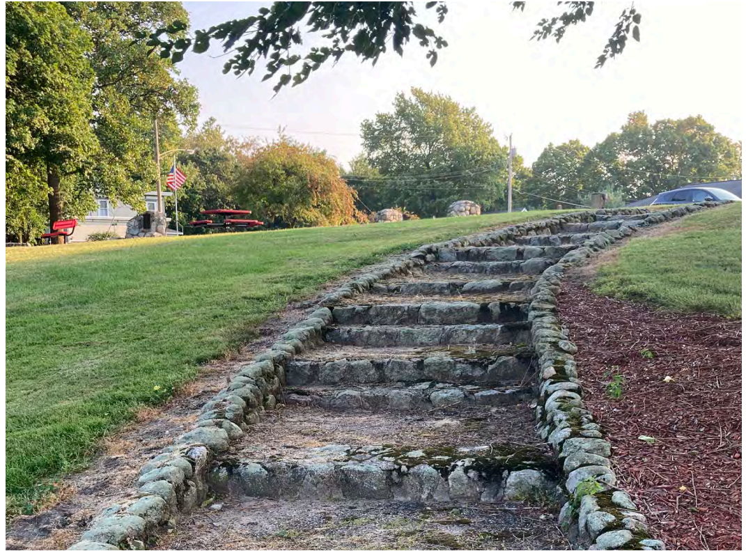
Stone Stairs in Town Park, While Historic can Be a Barrier For Users with Limited Mobility
