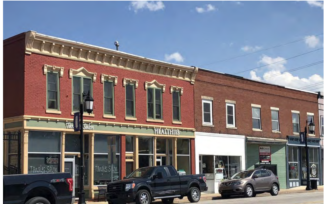
Storefront Facade Renovations
