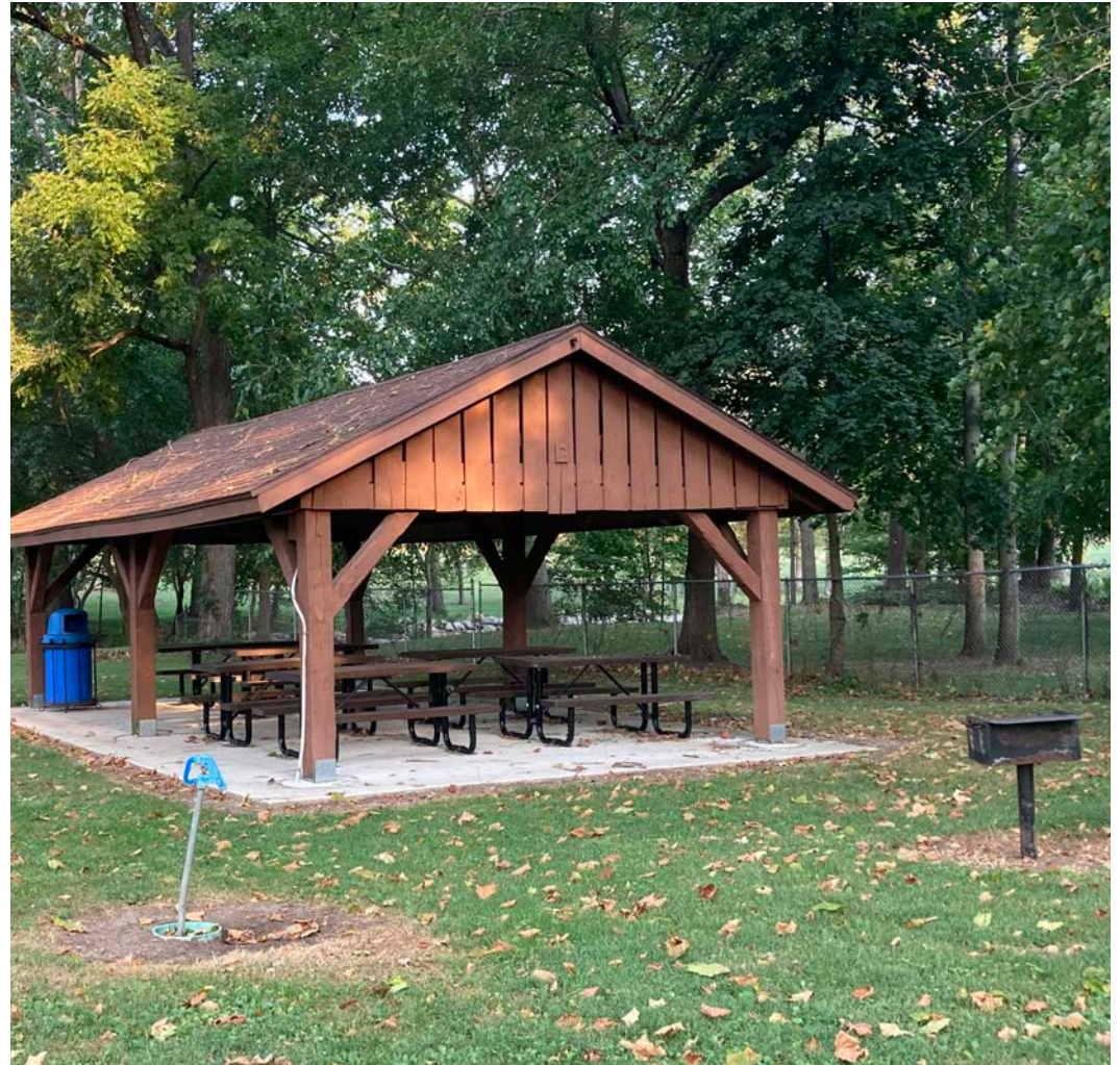
North Liberty Town Park, Picnic Shelter
