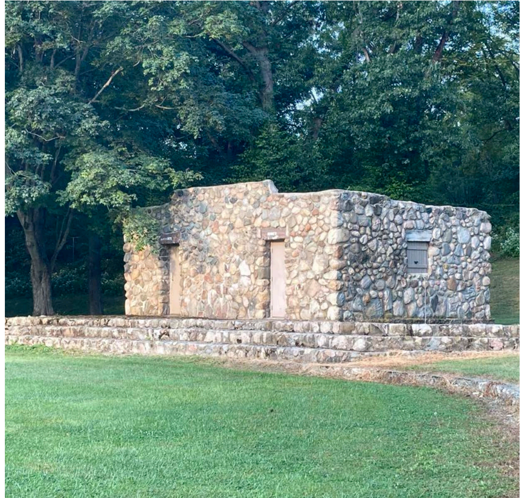
North Liberty Town Park, Restrooms
