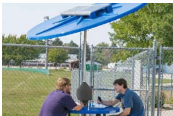
Solar Charging Station and Shade Structure (in process)
