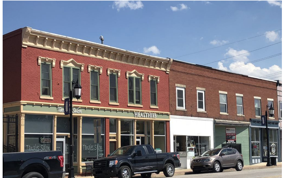
Storefront Facade Renovations
